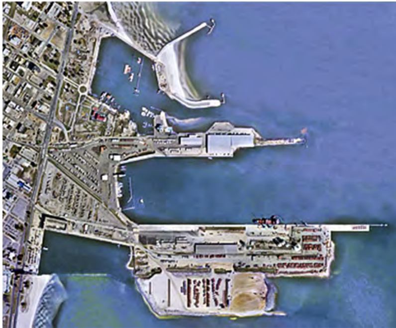
Fig. 5. Aerial view of Port of Gulfport ( www.portofthefuture.com ).
