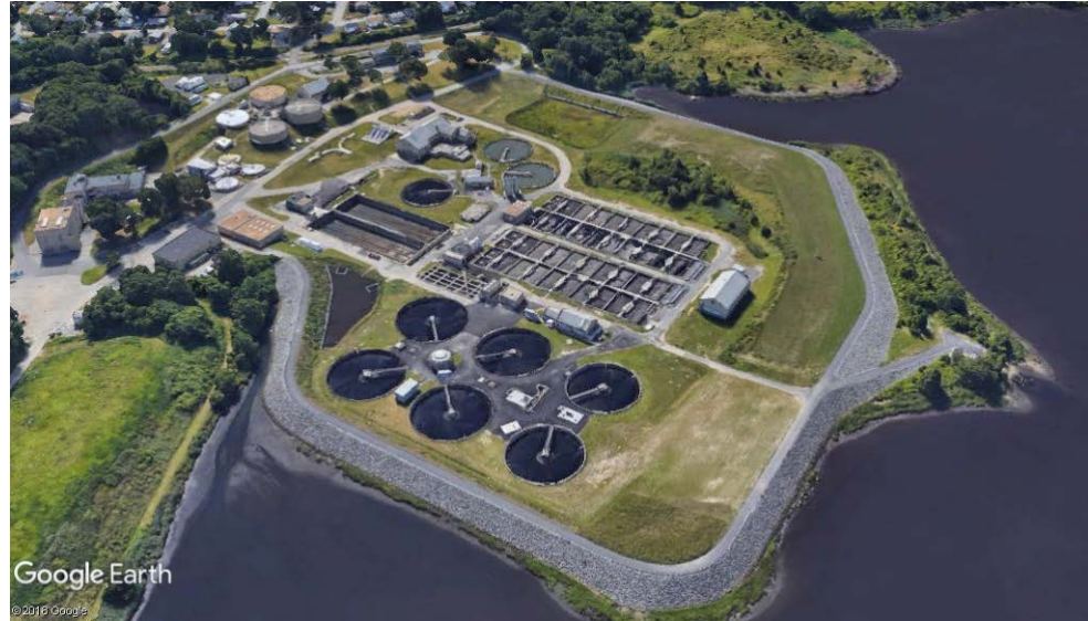
Bucklin Point Wastewater Treatment Facility
