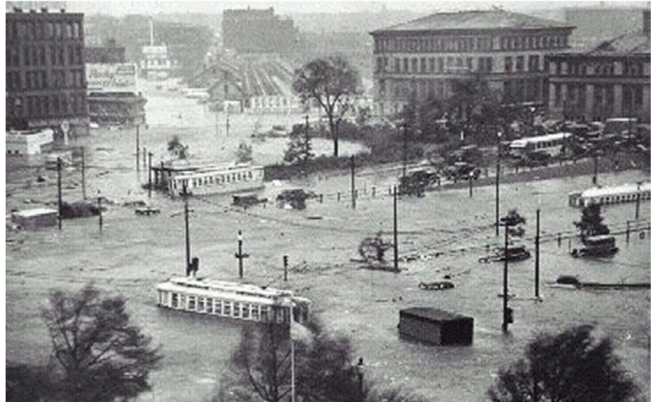
Flooding from the 1938 Hurricane in downtown Providence.
