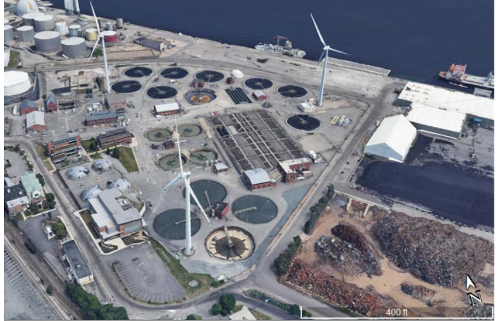
Fields Point Wastewater Treatment Facility
