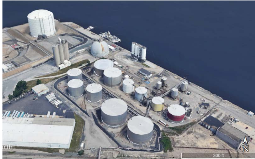
Above Ground Storage Tanks near Fields Point
