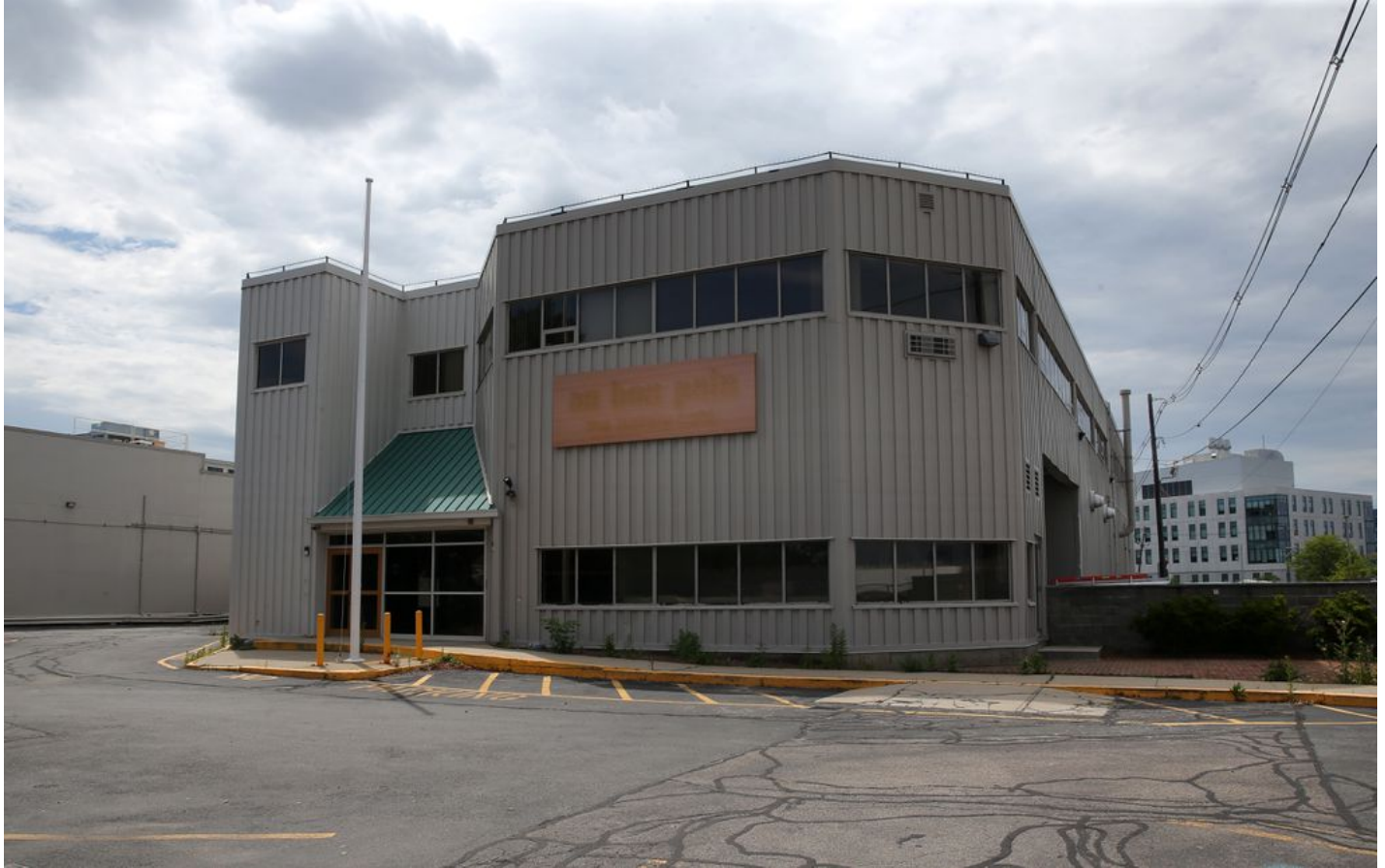
A view of the former Au Bon Pain headquarters in the Raymond L. Flynn Marine Industrial Park. DAVID L. RYAN/GLOBE STAFF
