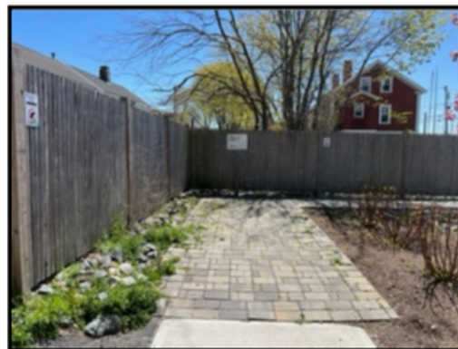
Exhibit 21: Abrupt and Unmarked Walkway Ending
