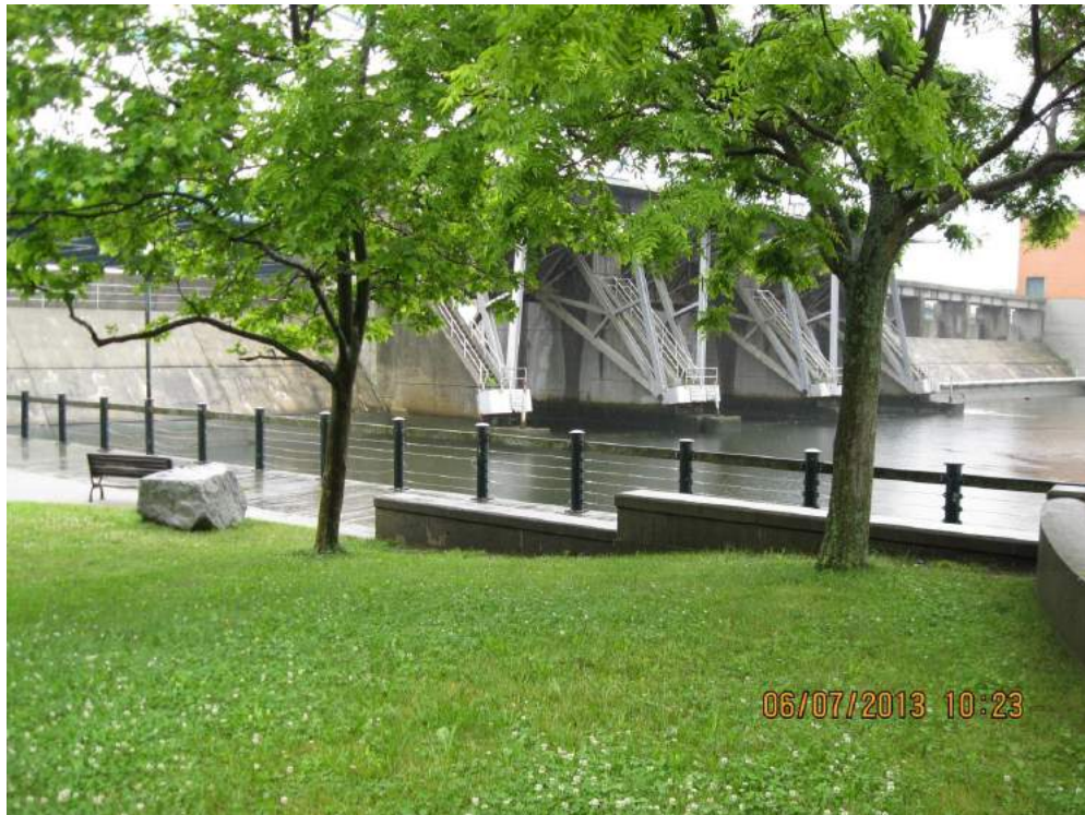
Harbor View Trail at the Fox Point Hurricane Barrier
