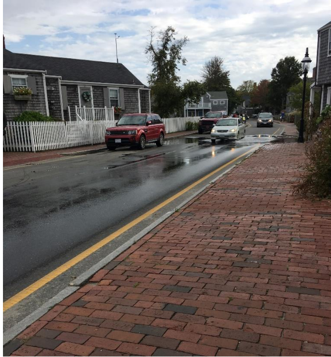
Figure 1, High-tide flooding on Easy Street at Oak Street on 10/2/2019 (15:55 local time) 1
