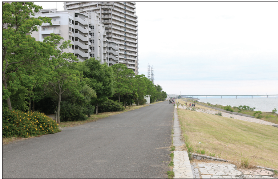
Figure 3. A superdike. This fixed landform is innovative because, unlike most earthen dikes, it is designed to allow buildings and trees to be built on the top level and on its back terraces. This gives residents a water view, increasing property values as well as raising awareness of the dynamic environment that surrounds them. This superdike was built in Osaka, Japan; it gains its unique structural qualities from being much wider (approximately 1200 ft) than a normal dike, which might be 400 ft wide to support 30 ft of height.
