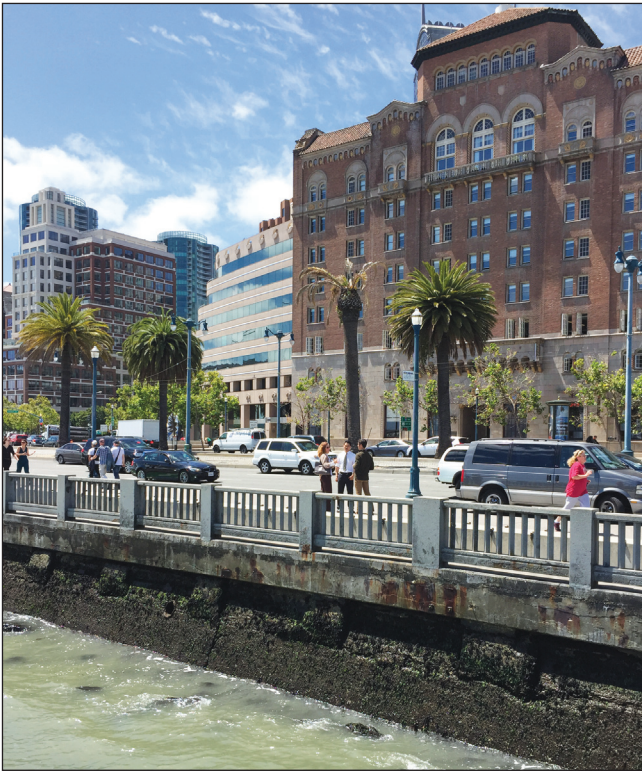
Figure 1. Seawall in San Francisco, California. Seawalls are fixed walls made of reinforced concrete or steel, often combined with wooden pilings treated with creosote. They are designed to retain unconsolidated fill on the landward side, which contains the footings of buildings and other infrastructure. Relieving platforms constructed of wood, or concrete and steel, hold the walls in place. These walls were essential for bringing ships directly into urban quays to efficiently load and unload cargo or passengers.
