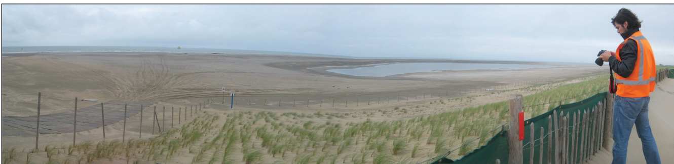
Figure 4. The Sand Engine. This 128-ha dynamic landform was built using 21 million cubic meters of dredged sand on the Dutch coast near The Hague in 2010. If it performs as designed, it will add 200 ha of beach along 10–20 km of coastline over 20 years as a result of wind and wave action, while adding habitat and recreational value (Stive et al. 2013). The dredged sand delta is intended to erode, feeding beaches and dunes up and down the ocean coast. If it is successful, more sand may be placed in this location to continue the strategy of mega-nourishment for the Dutch coast. This panoramic view from 2012 was taken from the dunes on the landward side of the Sand Engine, looking toward the sea.
