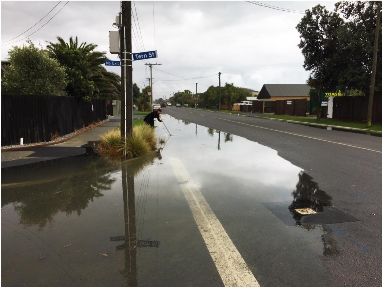
Figure 10. A woman tries to clear a storm drain on Tern Street during the high tide event. As groundwater rises, drain inlets like this one will be filled and will not drain unless special flaps are installed on the ocean outlet of drain pipes, and unless pipes are replaced when they crack.
