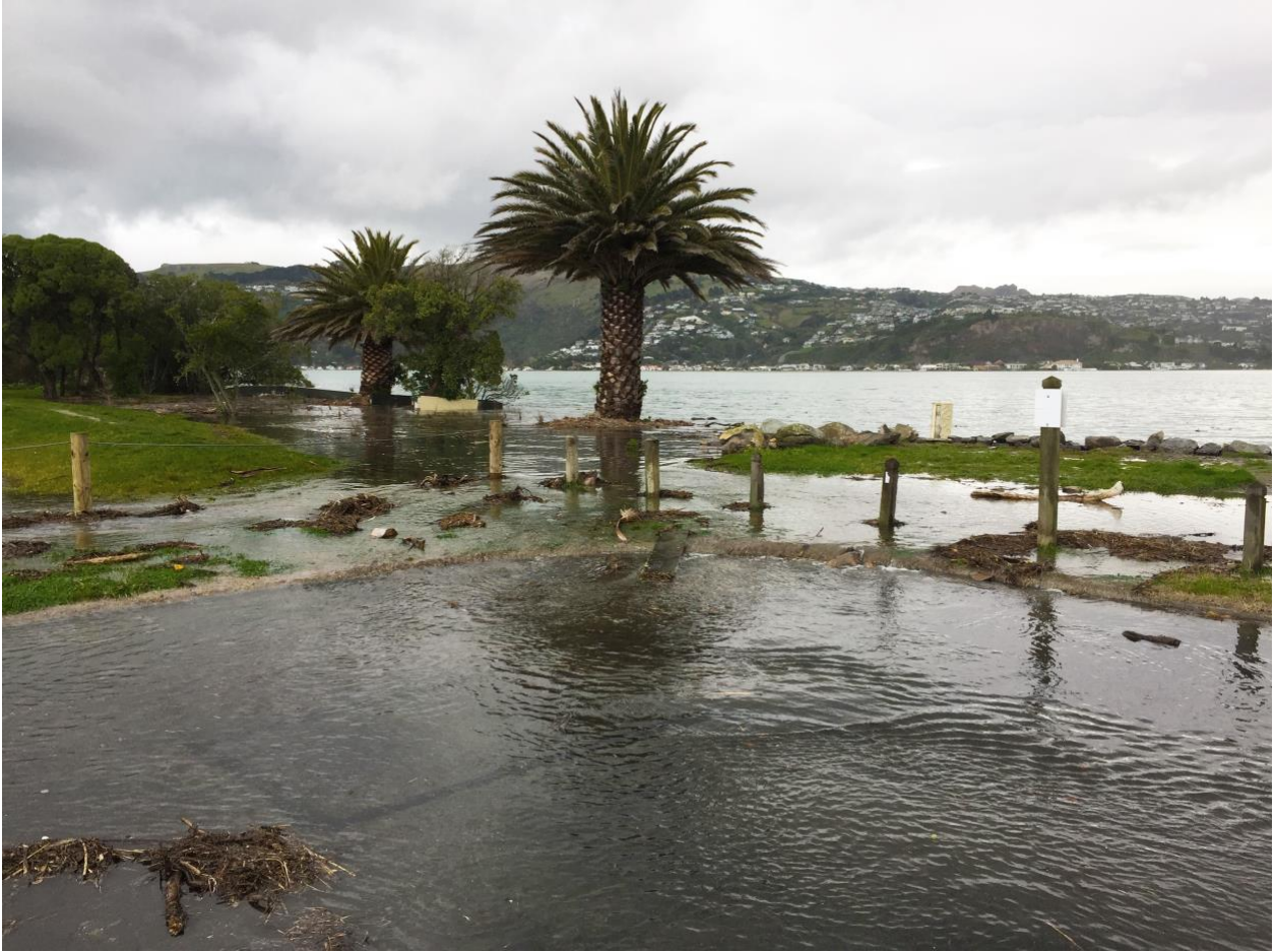
Figure 9. Flooding during an extra-high tide on Plover Street, Christchurch. Seawater from the estuary is flooding into the street, and being conveyed from there into the neighborhood.
