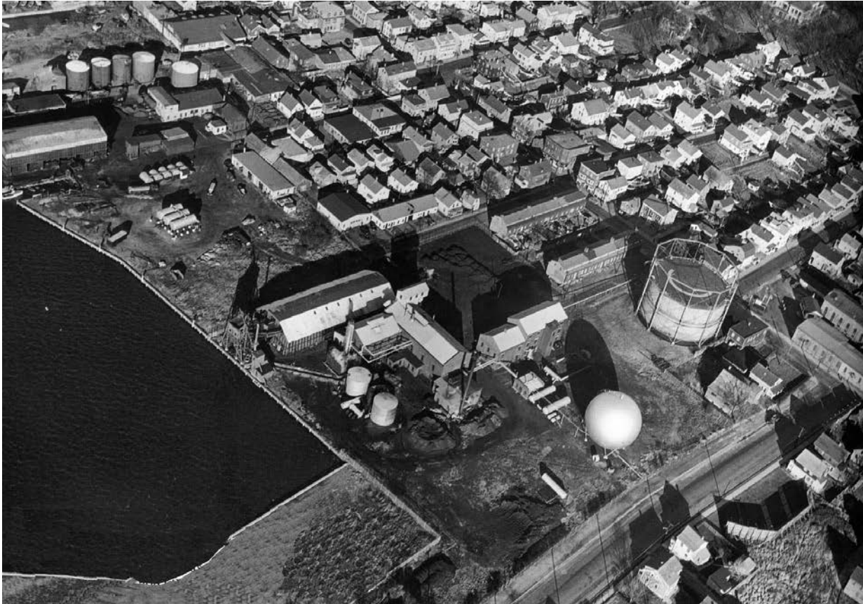
Figure 41: A ca. 1950's view of the Newport Gas Light Company. Notice the large 200,000c/f gasometer, coal bunker, retort house, and coke storage.
