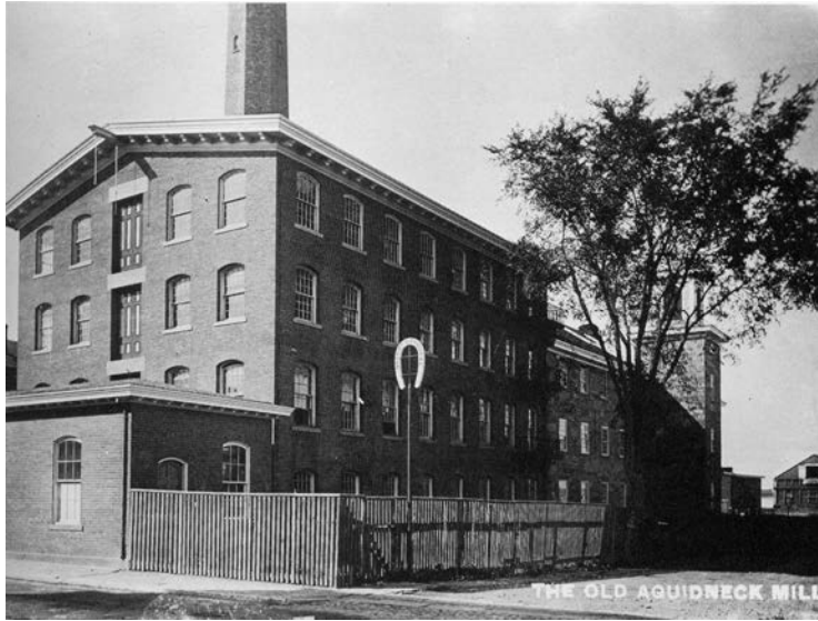
Figure 14: Aquidneck Mill c. 1880 showing belfry, 1865 addition and shot tower in background.
