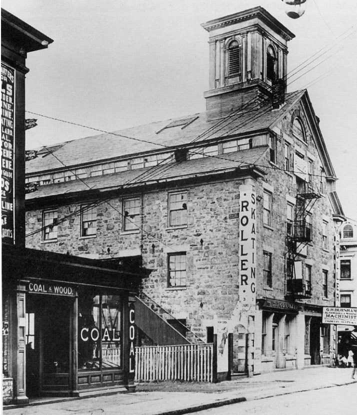
Figure 24: Perry Mill after c. 1913.
