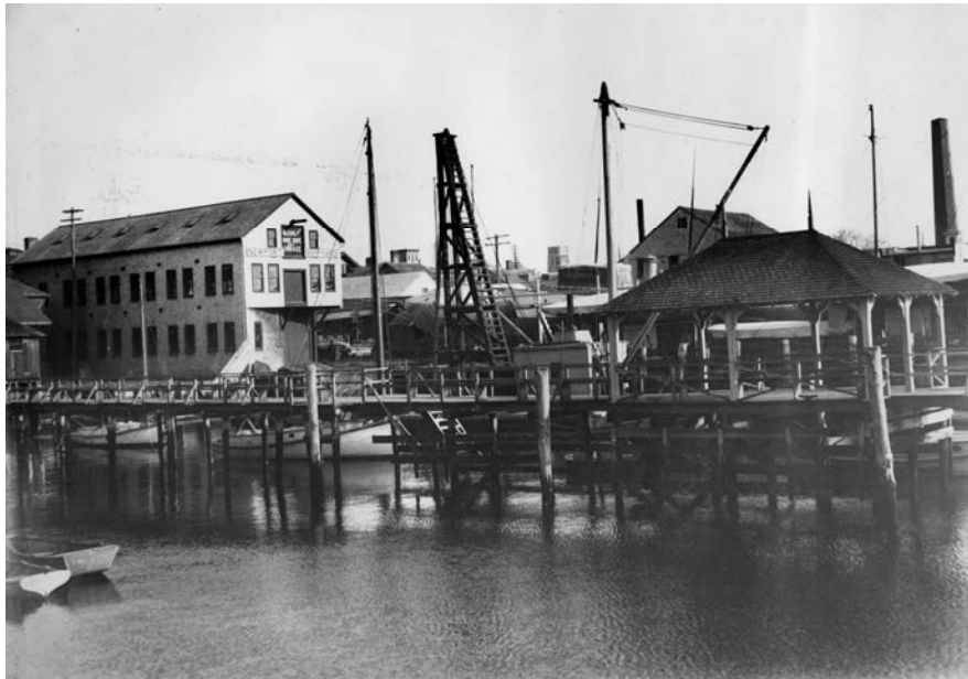
Figure 10: Newport Shipyard looking SE ca. 1920. Note Ann Street pier in foreground and large scissor behind that for pulling boilers/engines from ships. Shot tower for the Lead Works is on far right.
