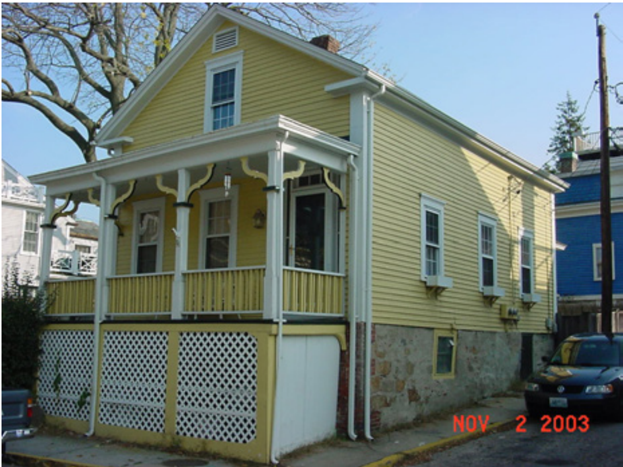
Figure 31: Potential tenement house (c. 1840) for the Richmond Manufacturing Company (Newport Steam Mill) at 360 Spring Street.
