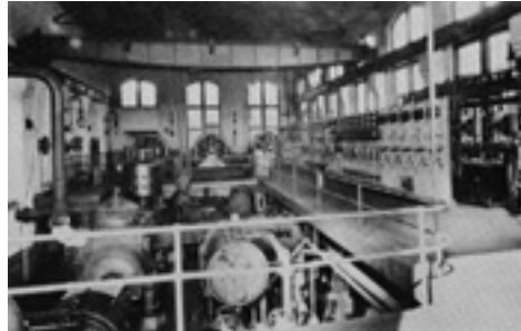
Figure 19: Interior showing 3 motor generators on far wall and turbo on left.
