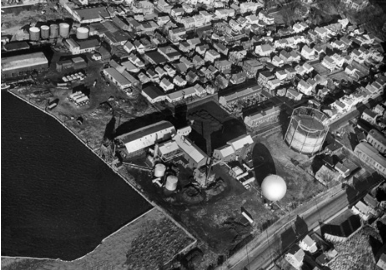
Figure 41: A ca. 1950's view of the Newport Gas Light Company. Notice the large 200,000c/f gasometer, coal bunker, retort house, and coke storage.
