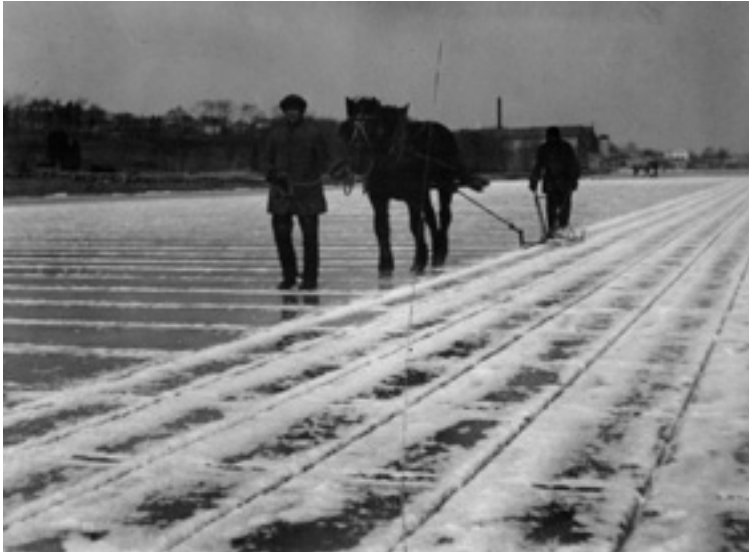
Figure 49: Cutting ice on Green End Pond with the Newport Ice Company ice house in the background.
