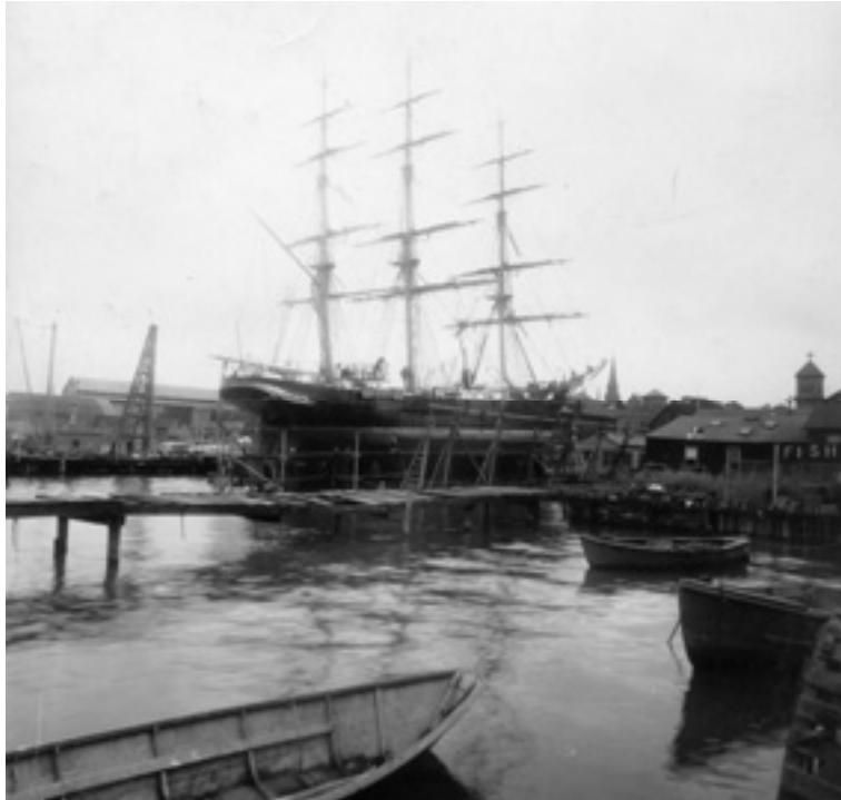
Figure 8: Newport Shipyard ca. 1920. Note ship on marine railway and condition of docks.
