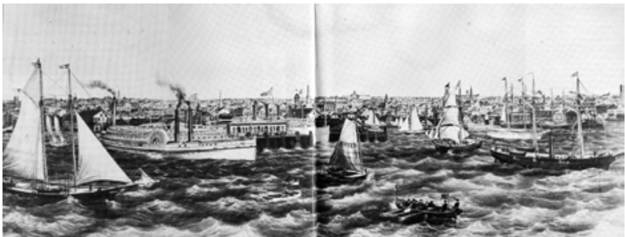
Figure 48: View of Long Wharf to Shot Tower, ca. 1870 (Newell).
