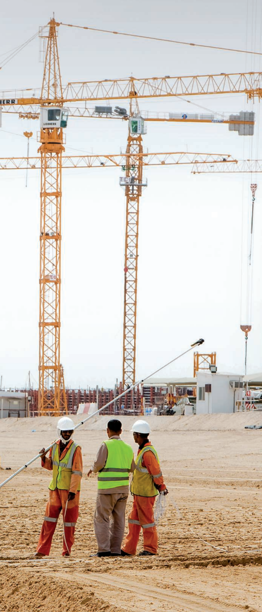
Workers engage in coastal construction in Dubai. Climate services technology is increasingly utilized to manage investment and construction risks.
