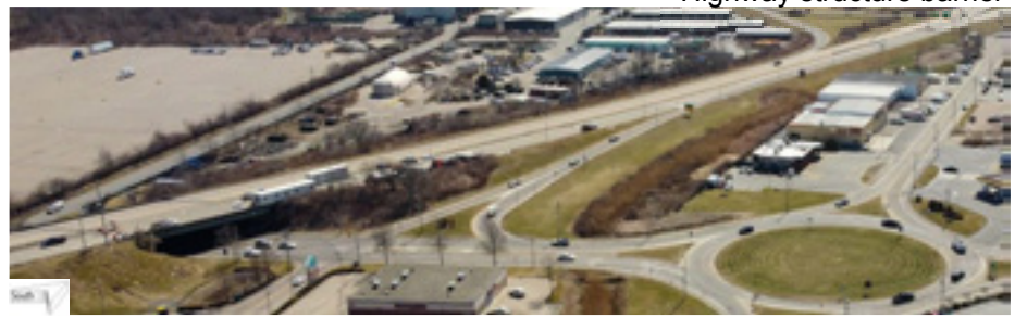
Highway structure barrier
