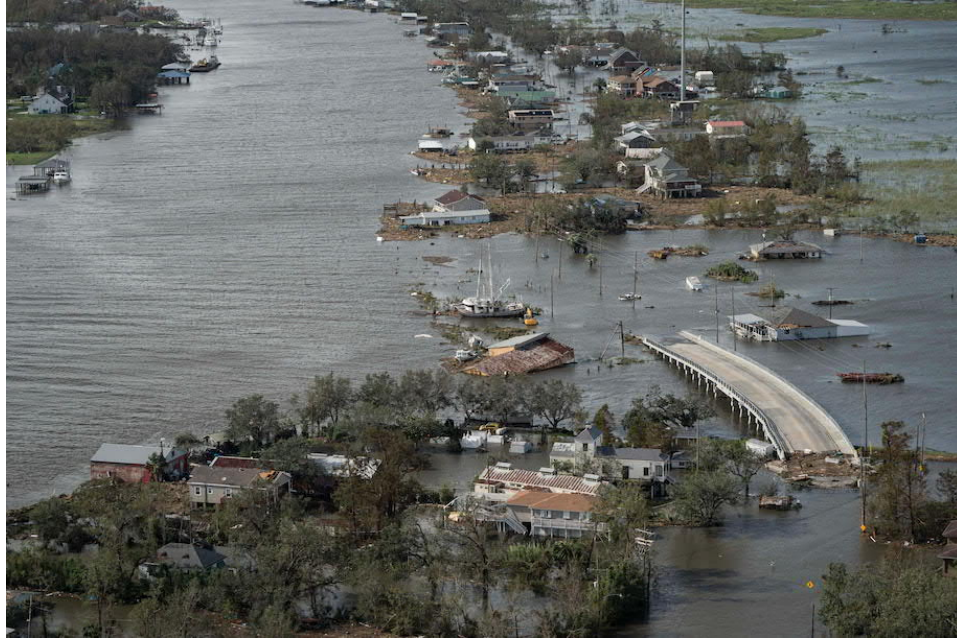
Figure 49. Flooding in Louisiana on August 30, 2021, caused by Hurricane Ida (Source: Washington Post)
