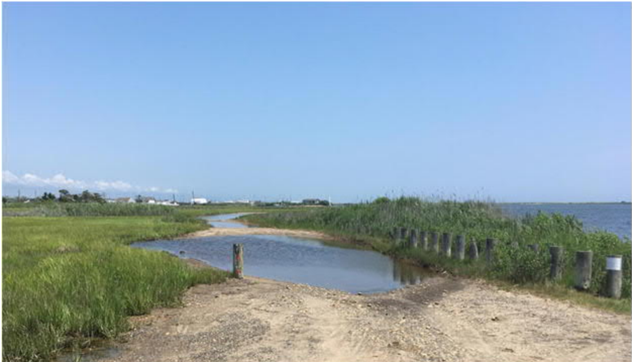
Figure 64. Image of Flooded Roadway at Mastic Beach
