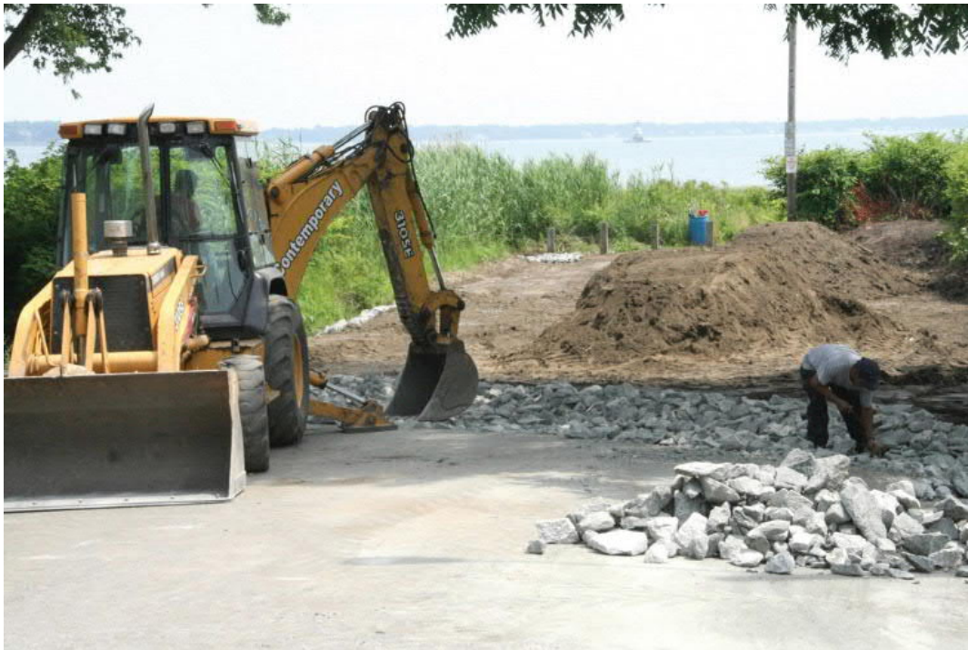
Figure 63. Image of End of Road Retrofit Construction on Mill Cove Road
