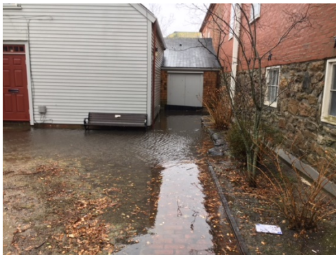
Gift Shop & Connector north Elevation. Photos taken during the flood illustrate the major pathway of the January 4 th flood waters into the building were through the Connector exit doors seen in the photo on the left. The photo of the open area to the north of the Gift Shop illustrates the concurrent need to regrade this area to provide positive drainage to the east. Photo credit: Ed Rudd
