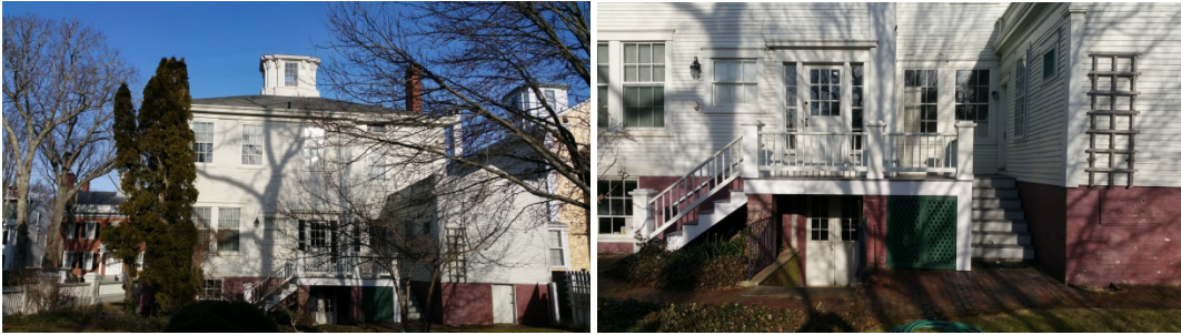
Photo Rear Elevation of the Hadwen House – Developing an appropriate architectural plan for the addition of an elevator and ADA accessible ramp to the rear deck (first floor) level of the Hadwen house for this character defining exterior elevation will be a challenge. The accessibility enhancement must be designed so that the exterior appearance of this NHL home is not diminished.
