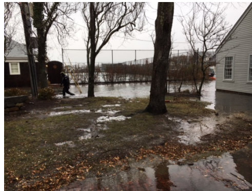
Gift Shop & Connector north Elevation. Photos taken during the flood illustrate the major pathway of the January 4 th flood waters into the building were through the Connector exit doors seen in the photo on the left. The photo of the open area to the north of the Gift Shop illustrates the concurrent need to regrade this area to provide positive drainage to the east. Photo credit: Ed Rudd
