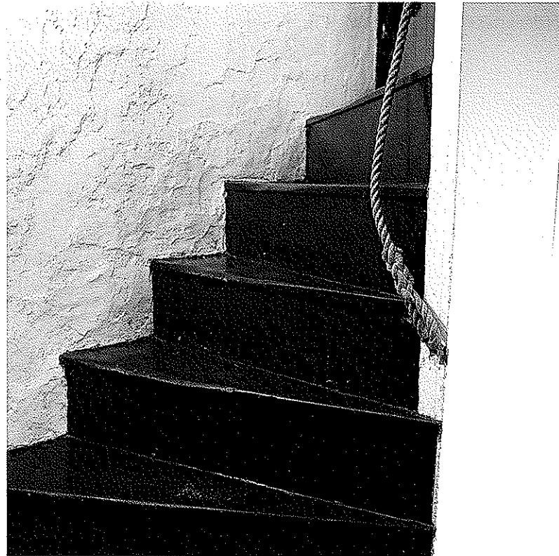
Stairwell with Rope Handrail.
