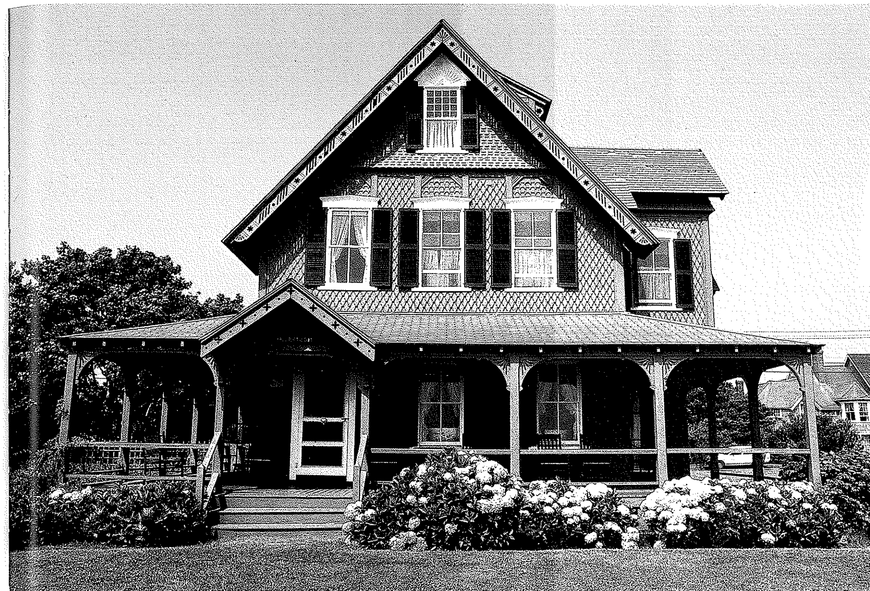
FIGURE 15: Idlemoor, Built in 1884, 11 Baxter Road, ‘Sconset. Victorian architecture by nature is inventive and diverse in color and style, as can be seen in the rich blue color, fanciful trim, and decorative shingle work of Idlemoor. On a bright, sunny day, the vergerboards enliven the facade by creating a lively pattern of shadows across the surface. Photograph by Gregory Spaid.
