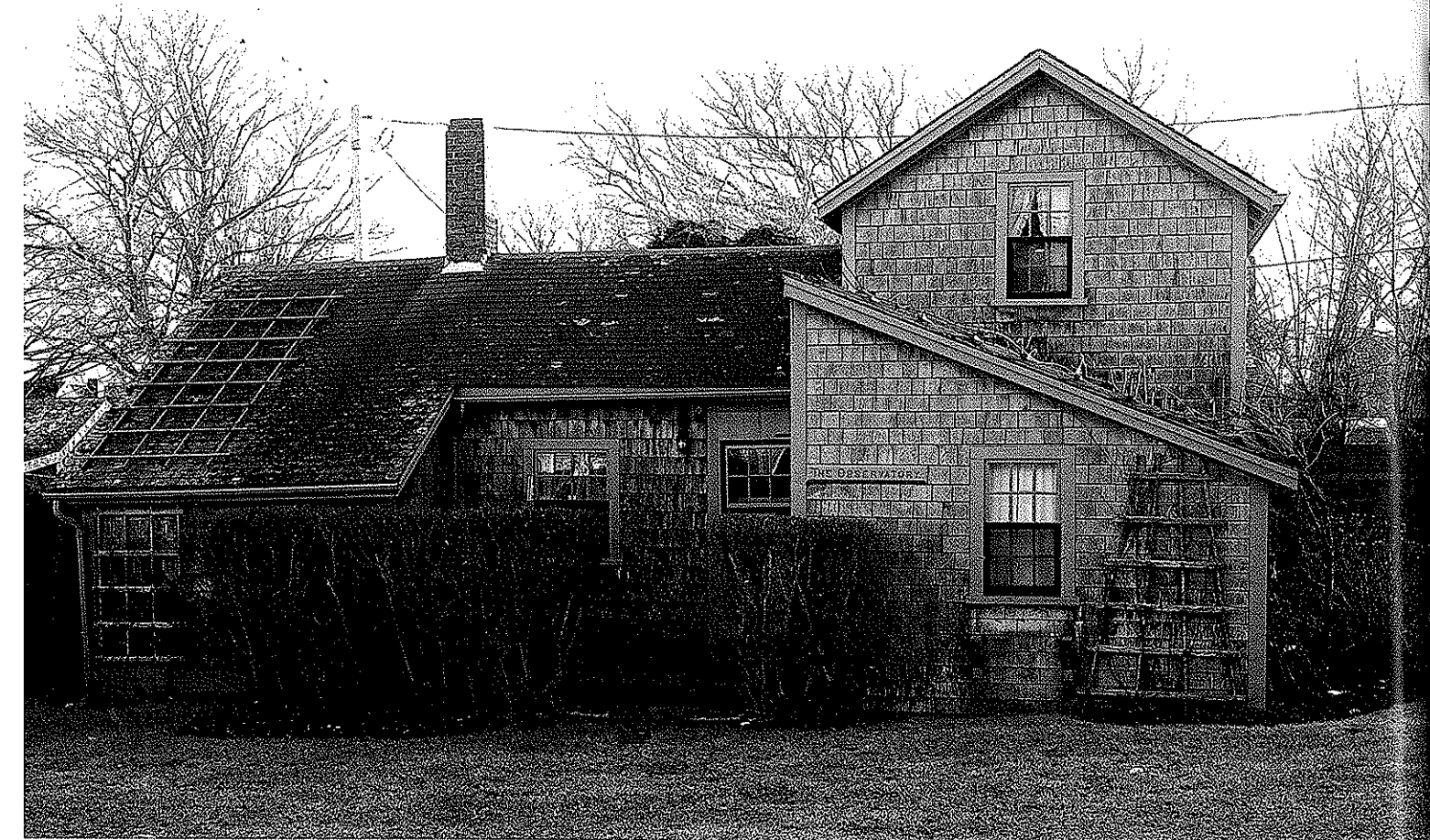
FIGURE 20: The Observatory, Built ca. 1888–89, 6 Lily Street. The one-story shed roof front projection, which can be seen in this cottage, is said to be called a “flounder.” The wedged-shaped form was adapted by Edward Underhill from additions found on the whale houses, specifically in the cottage known as “The Corners,” located near the former Sconset water pump.
