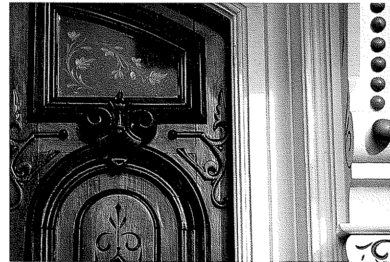
FIGURE 3: Detail of the Door at 73 Main Street. With its exquisitely carved wood and etched-glass panel, this door reflects the Victorians’ belief that the first and most important impression made upon a visitor to a house was through its entranceway.
