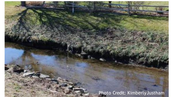
stormwater runoff moat encircling south pond
