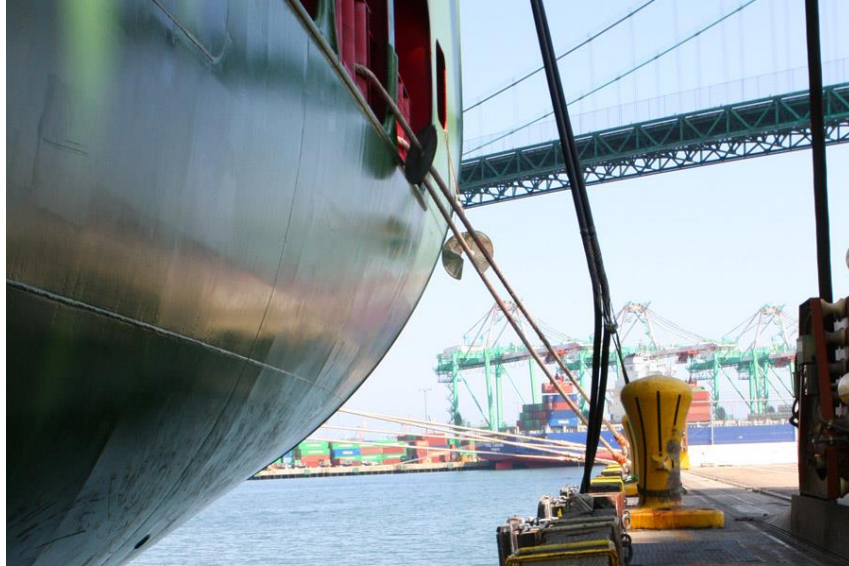
Figure 6: The Port of Los Angeles- Shore Power
