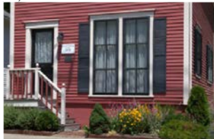
Appropriate The material used for the stairs is consistent with the foundation material.
