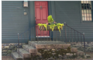
Appropriate The material used for the stairs is consistent with the foundation material.
