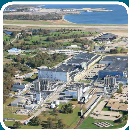
Toray cogeneration facilities
