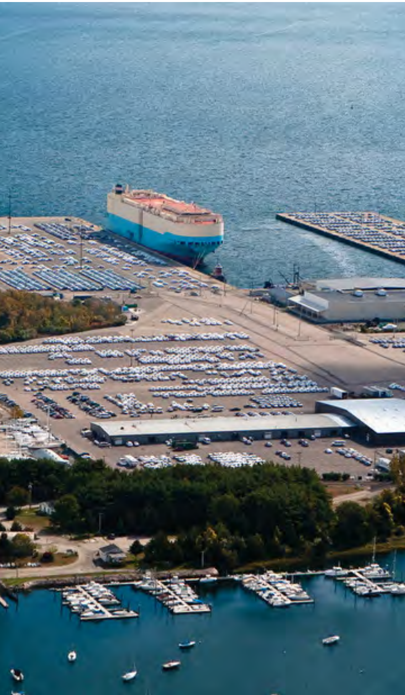
Port of Davisville in Quonset Business Park.
