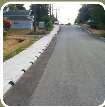
At-grade curb separated walkway
