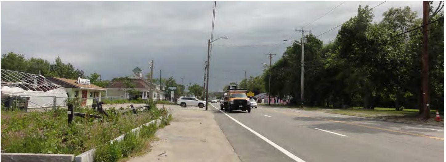
South Post Road has no sidewalks or crosswalks. With no turning lane, cars turning left to access businesses increase the risk of rear end collisions. The stretch between Huling Road and Camp Avenue is particularly dangerous, accounting for 30% of the crashes along Post Road between 2008 and 2015.
